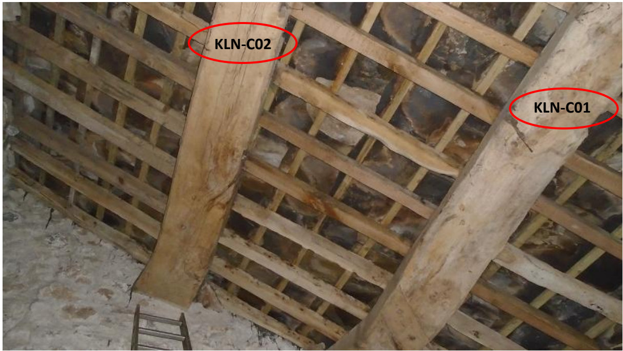
Figure 2: Annotated photograph to help identify sampled timbers
